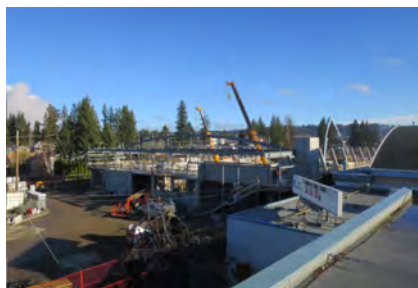
Figure 7 City of Quesnel's new West Fraser Centre Arena
