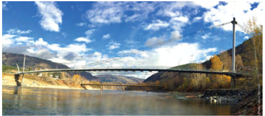
Figure 6 The new Columbia River Skywalk in Trail
