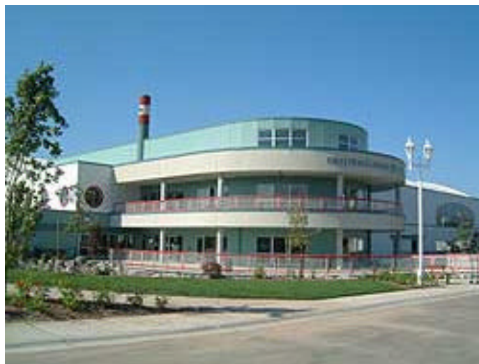
Chilliwack Landing Leisure Centre
