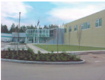
Oceanside Place Multiplex Arena
